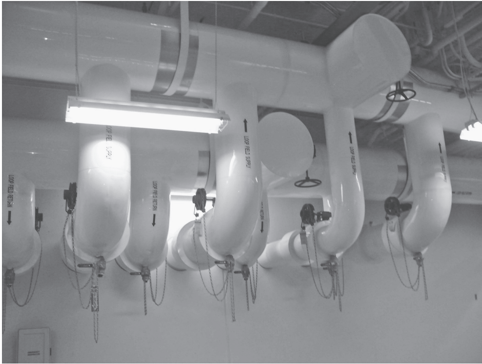
Fig. 14.139 Supply and return well field water headers at the energy stations. (© Ball State University; Reproduced and reprinted under license from Ball State University. All rights reserved.)
