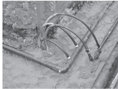
Fig. 14.138 Borehole wellhead showing the 6 in. (152 mm) diameter HDPE closed-loop tubing. (© Ball State University; Reproduced and reprinted under license from Ball State University. All rights reserved.)
