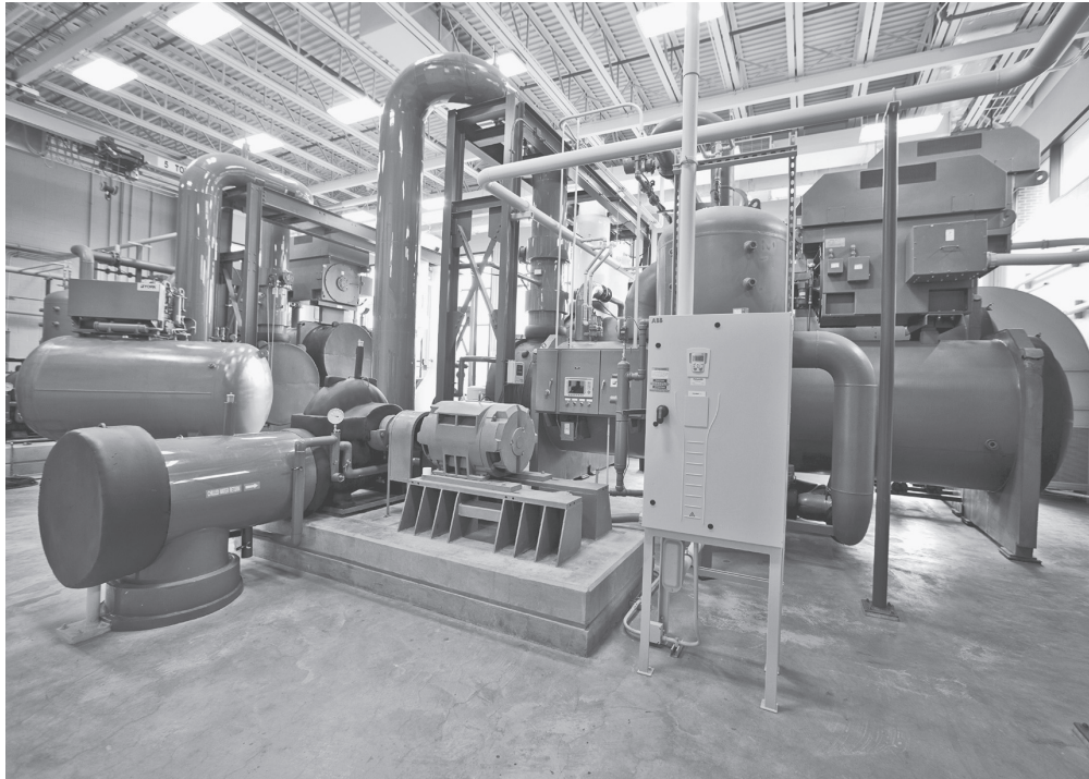
Fig. 14.140 One of four 2500-ton (8790 kW) heat pump chillers used at the district energy stations on campus. (© Ball State University; Reproduced and reprinted under license from Ball State University. All rights reserved.)
